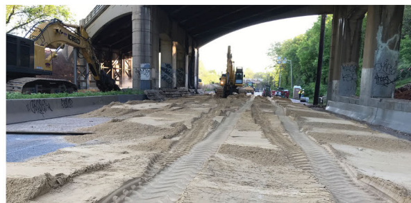
Sand Protecting MD 295 During Annapolis Road Bridge Demolition
